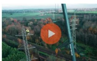
The new line running between Harchies and Quevaucamps in Belgium has been completed following two years of work that involved the route being optimised and the pylons and conductors being replaced. The works began at the end of March 2021 and covered a 5.4 kilometre section of the line. The old section of the line had been built in the 1960s, meaning that in 2021, the conductors no longer matched current standards. The new section of line was constructed before the old one was dismantled.
