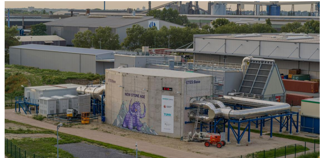
Siemens ETES in Hamburg: 1000 t rock, 6 MW th /130 MWh th or 1,5 MW e /30 MWh e from steam turbine
