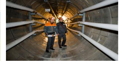
2. Berlin Cable Reinforcement 380-kV-Cable Berlin
