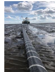
4. Nemo Link Subsea HVDC-interconnection with UK
