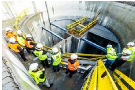
4. Nemo Link Subsea HVDC-interconnection with UK
