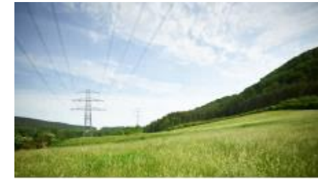
2. South-West interconnector 380 kV line crossing Thuringia
