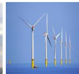
5. Ostwind 2 2nd Cluster Westlich Adlergrund / Offshore connection in the Eastern German Baltic shore
