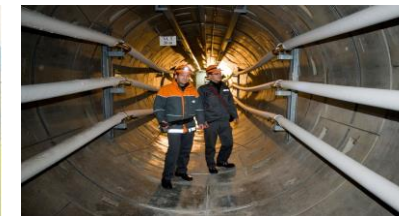
2. Berlin Cable Reinforcement 380-kV-Cable Berlin
