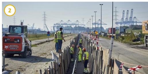
2 Brabo Strengthen the high-voltage grid and security of supply in the port of Antwerp and Belgium
