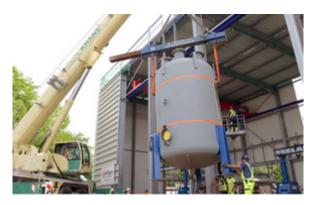
The two large electric boilers for the Power-to-Heat (P2H) project between Hamburger Energiewerke and 50Hertz have been successfully installed. By the end of this year, the P2H system must provide about 27,000 apartments with green city heating. The system converts electricity into heat when plenty of wind energy is available and grid congestion is imminent. 50Hertz is financing the 80 MW plant with €31.5 million.
